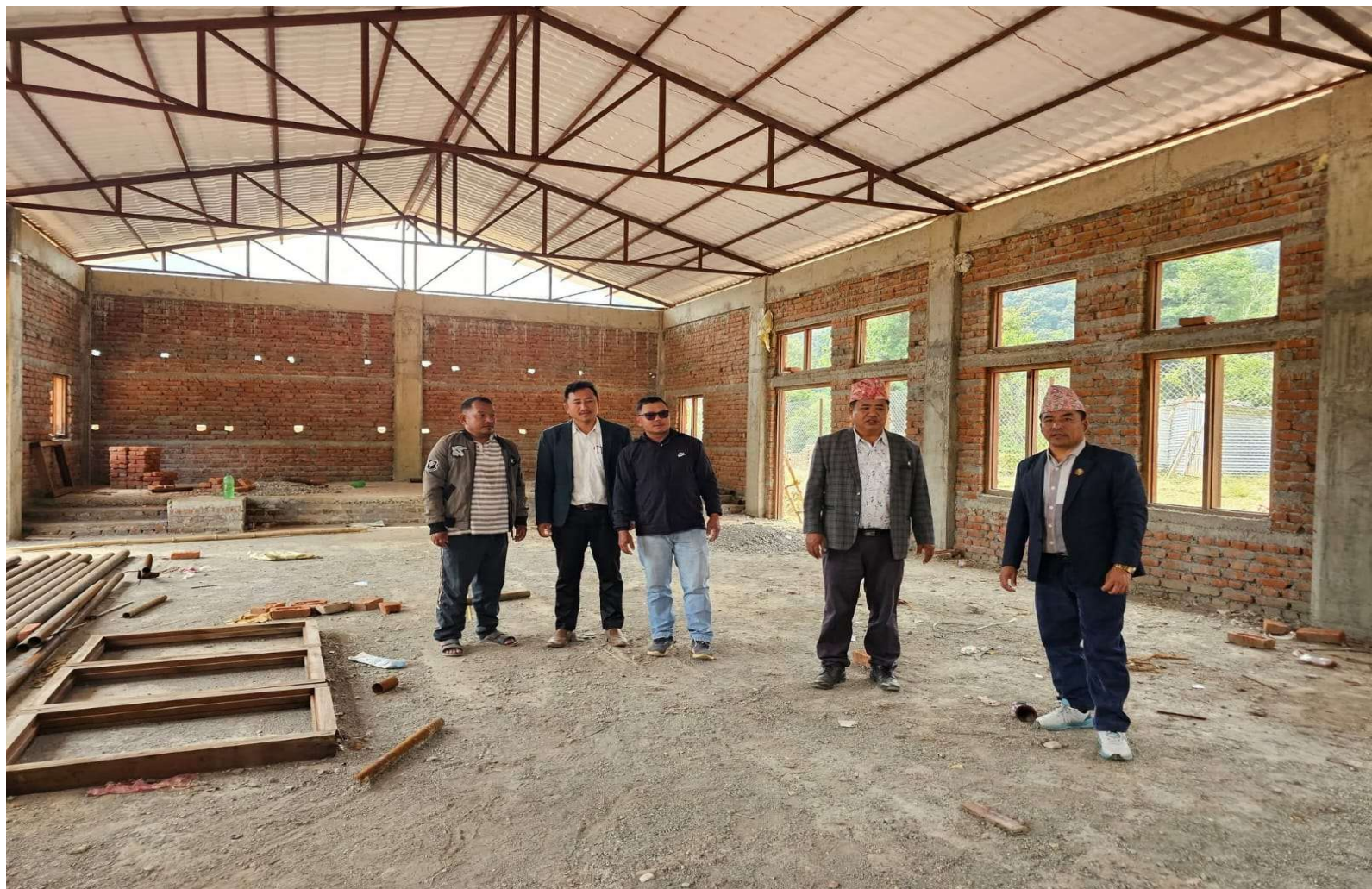
Administrative Building of Mathagadhi-04, Jhadewa, Palpa (Sabhahall)
