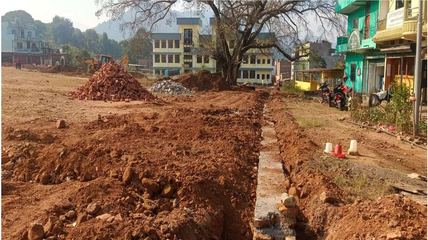
Construction of Canteen Block and Compound wall of Divyajyoti Secondary School-
