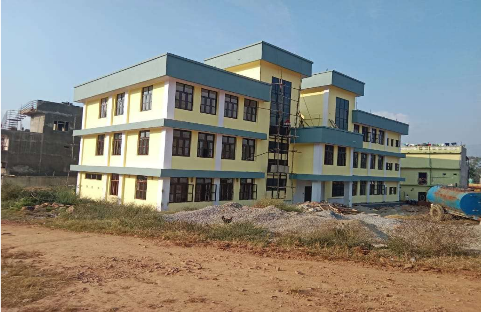
Divyajyoti Secondary School, Mathgadhi-03, Palpa
